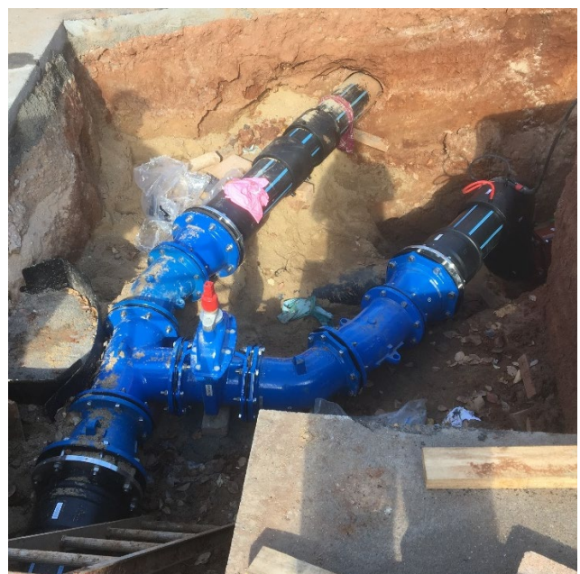
Hillston High Street, Mains Replacement
