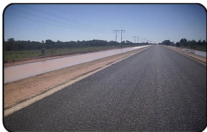
Carrathool Road, Pave and Seal – April 2020
