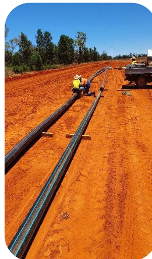
Langtree Mains Replacement
