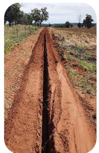
Melbergen Mains Replacement
