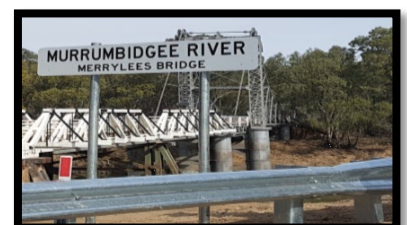
Carrathool Merrylees Bridge
