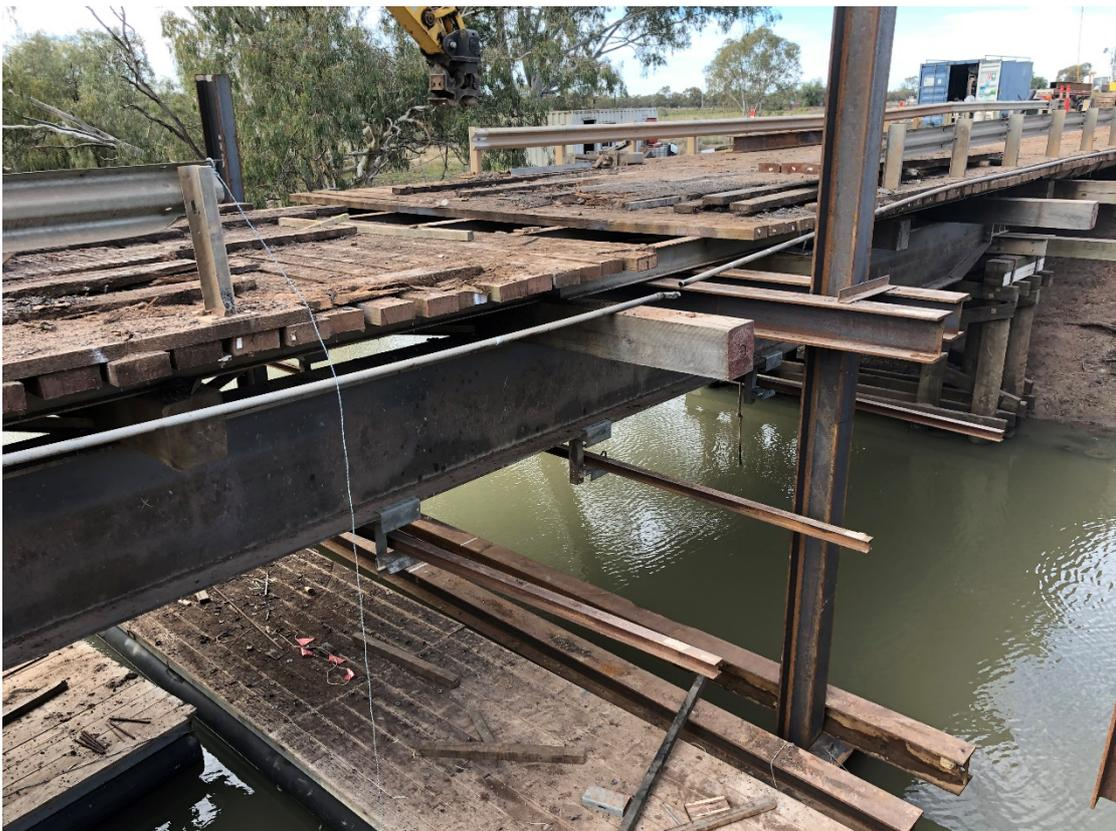
Photo 2 – Existing Bridge – Construction of Formwork for Piling
