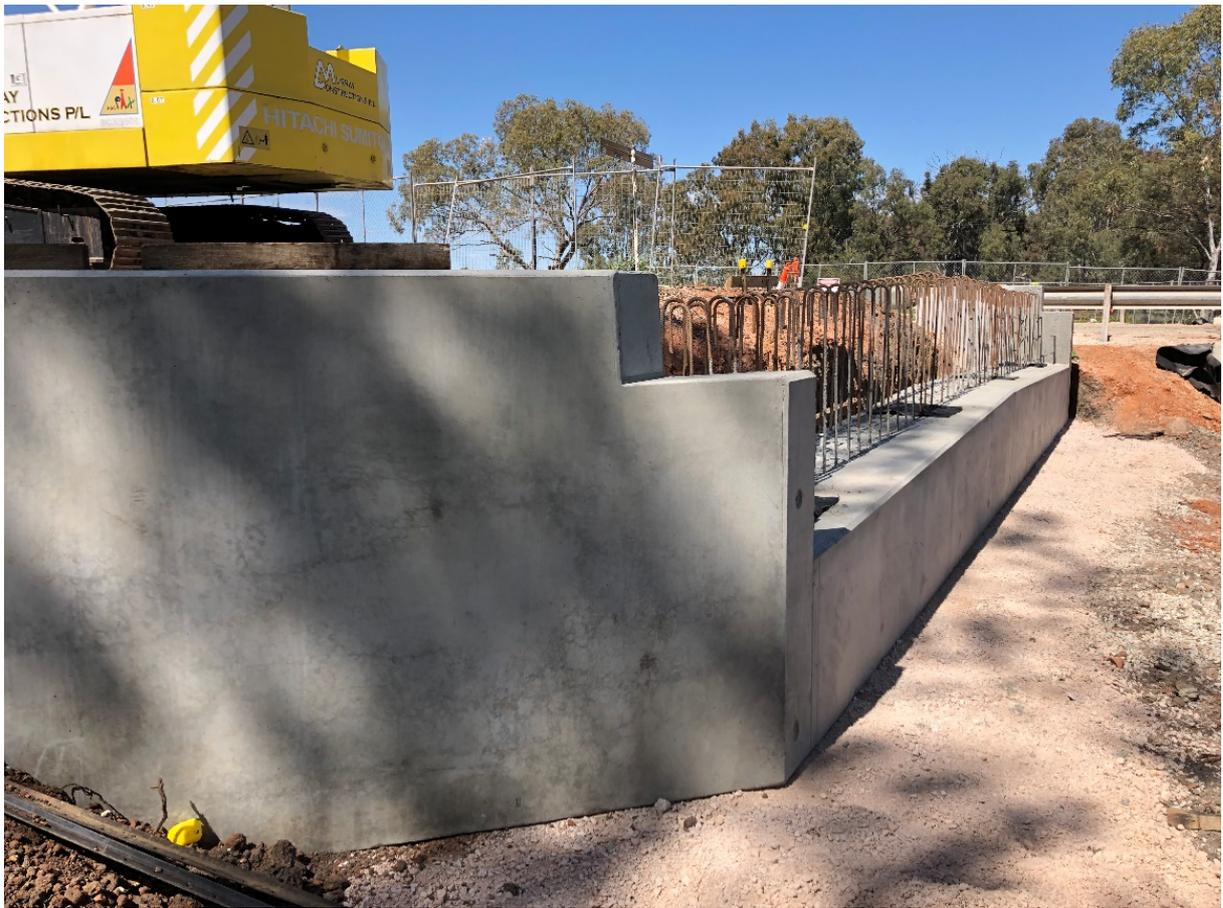
East Abutment – Precast Structure in Place and Anchored
