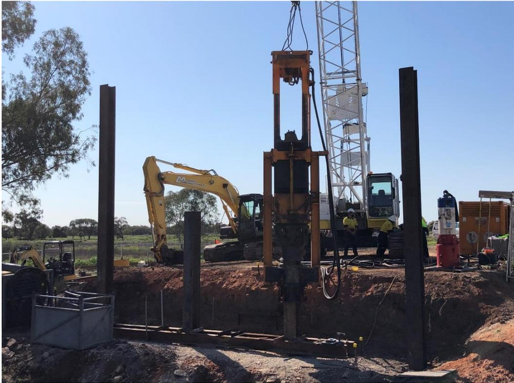
East Abutment – Construction of Formwork for Piling in Progress
