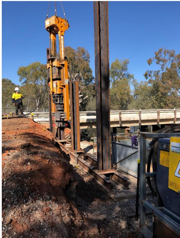
East Abutment - Pile Hammer in Action
