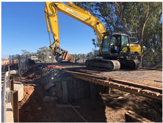
Photo 1 – Existing Bridge West Approach – Decommissioning in Progress
