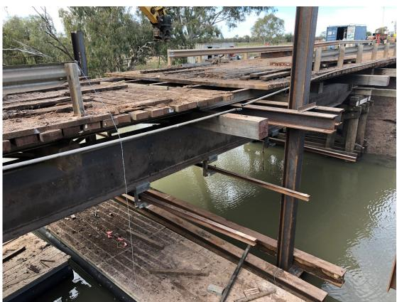
Photo 2 – Existing Bridge – Construction of Formwork for Piling
