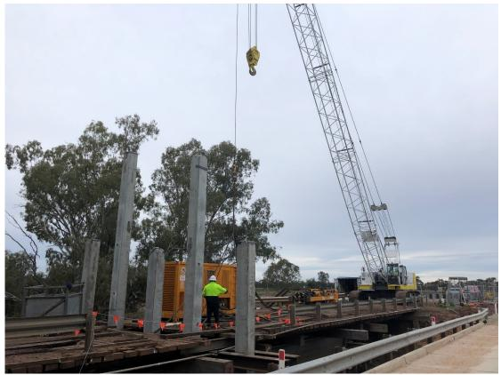
Photo 3 – Construction of Centre Piles in Progress
