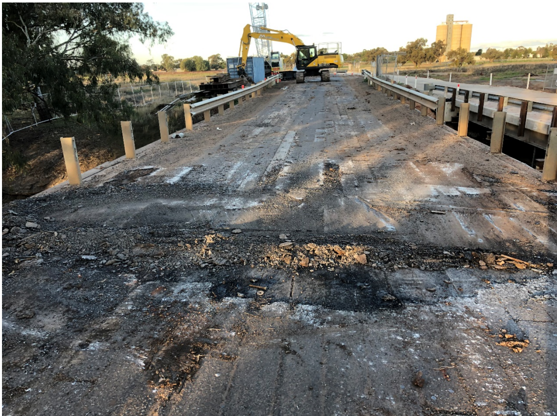
Photo 2 – Existing Bridge West Approach – Decommissioning in Progress
