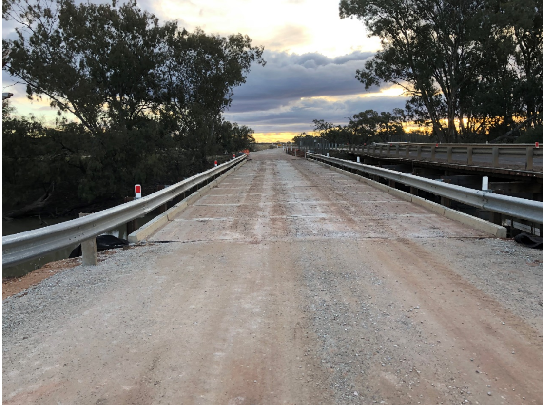
Photo 1 – Temp Bridge (Detour) – Complete & Operational
