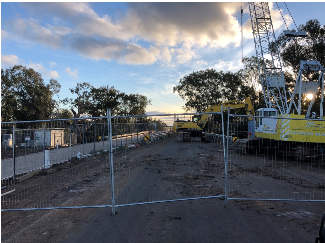
Photo 4 - Existing Bridge – Decommissioning in Progress
