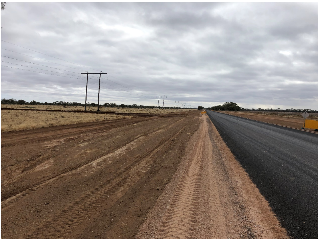
Photo 4 – Carrathool Road Construction – Stage 2
