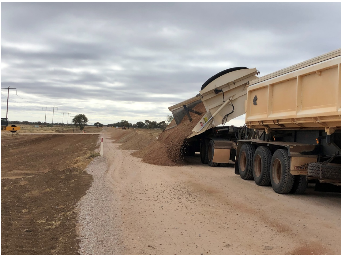
Photo 2 – Carrathool Road Construction – Stage 2
