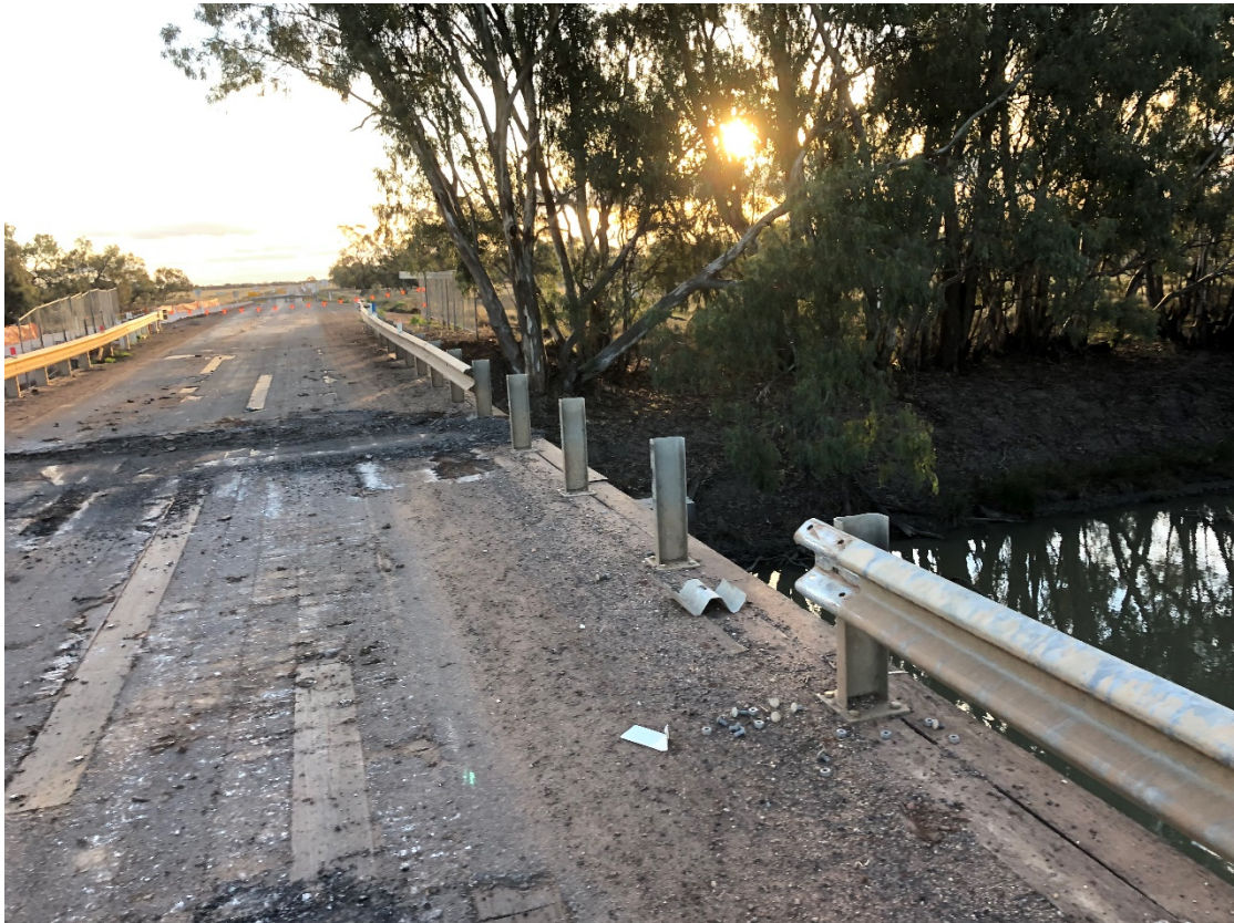
Photo 3 - Existing Bridge – Decommissioning in Progress
