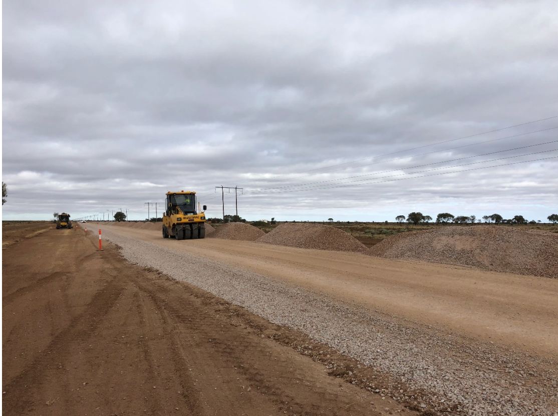
Photo 1 – Carrathool Road Construction – Stage 2
