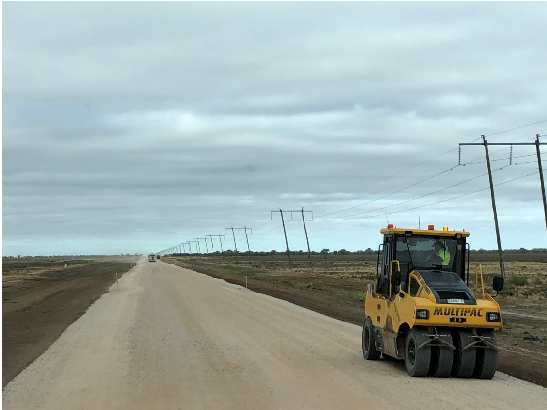
Photo 3 – Carrathool Road Construction – Stage 2
