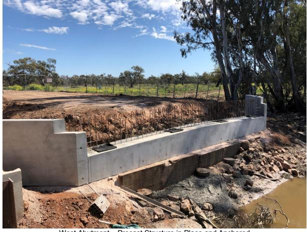
West Abutment - Precast Structure in Place and Anchored
