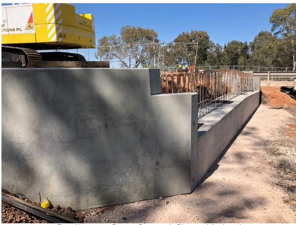
East Abutment - Precast Structure in Place and Anchored
