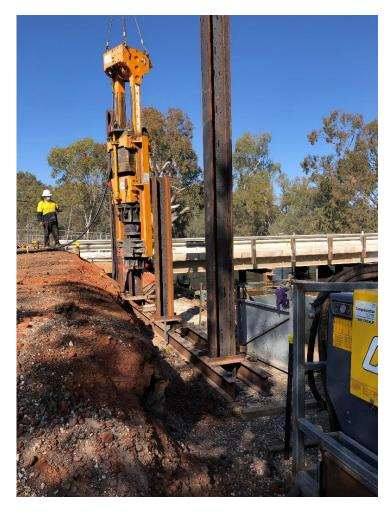
East Abutment - Pile Hammer in Action
