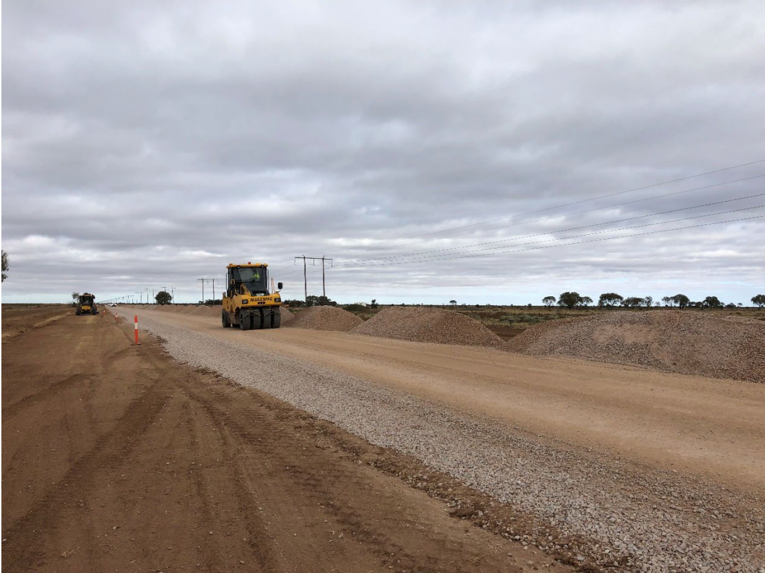
Carrathool Road Construction – Stage 2
