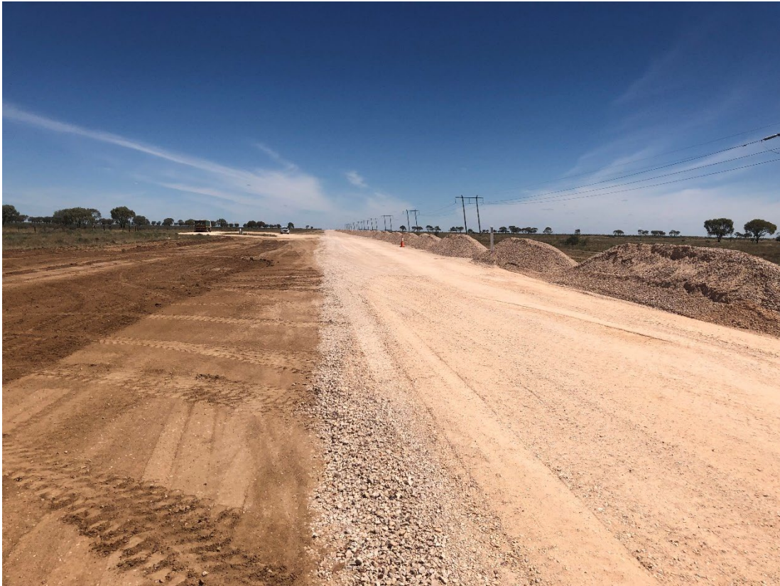
Carrathool Road Construction – Stage 3
