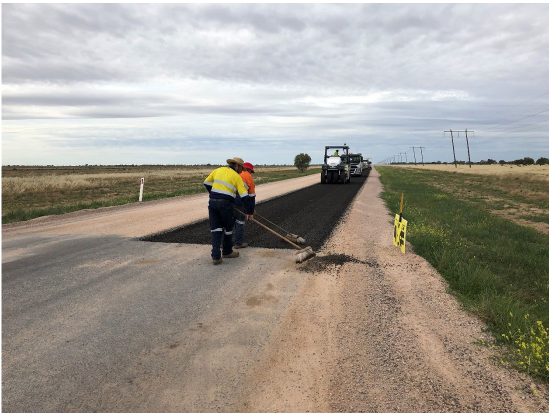
Carrathool Road Construction – Stage 3
