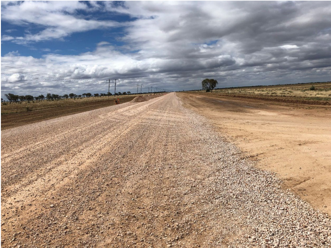
Carrathool Road Construction – Stage 3
