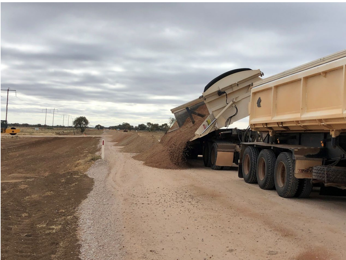
Carrathool Road Construction – Stage 2
