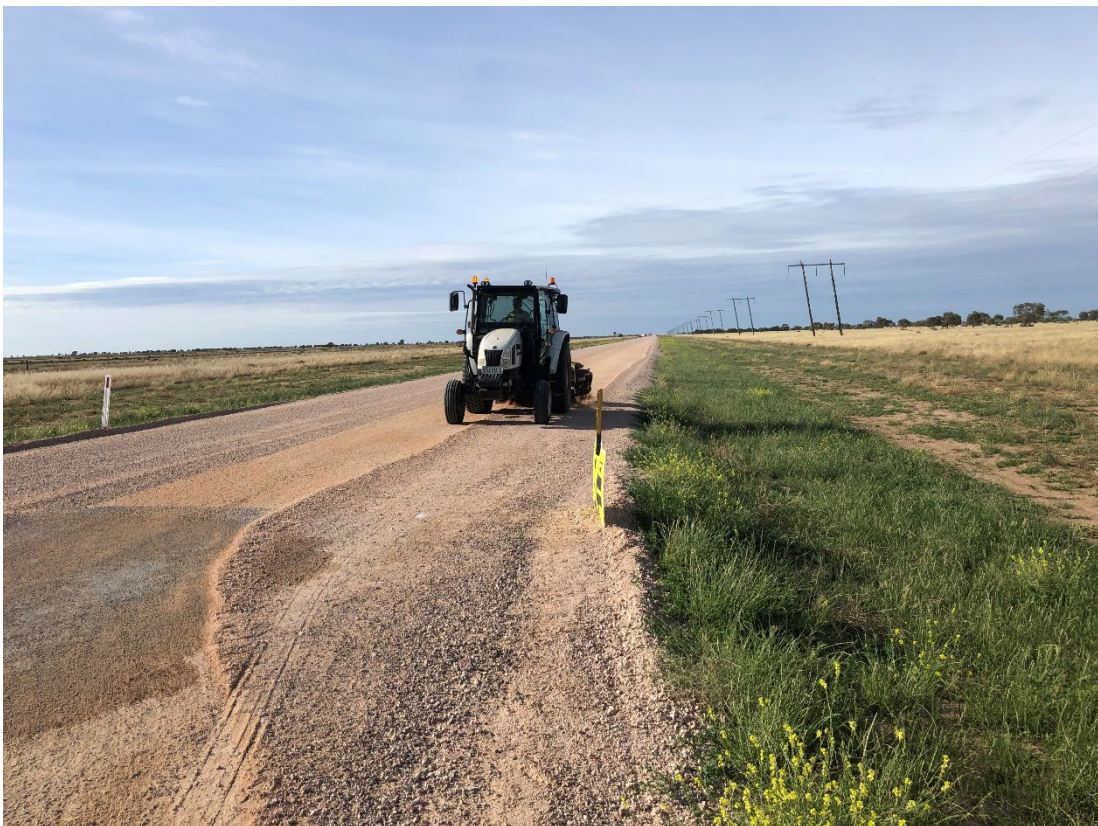
Carrathool Road Construction – Stage 3
