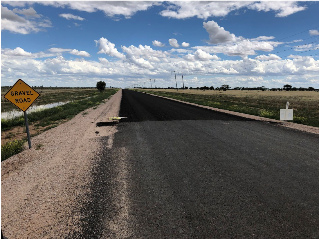
Carrathool Road Construction – Stage 3
