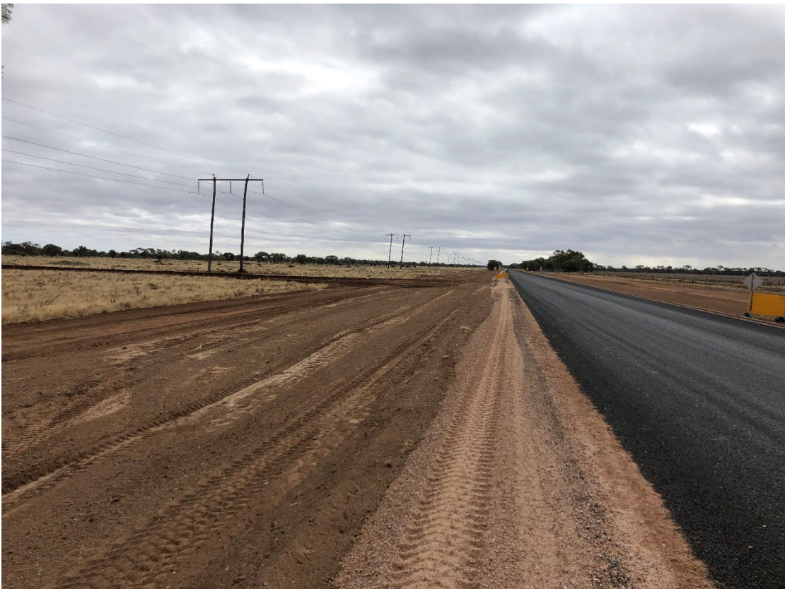
Carrathool Road Construction – Stage 2
