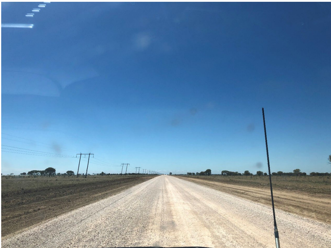
Carrathool Road Construction – Stage 3
