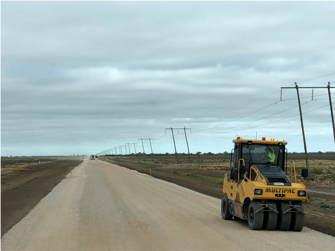
Carrathool Road Construction – Stage 2
