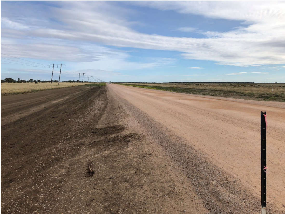
Carrathool Road Construction – Stage 3
