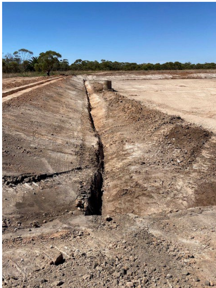
Goolgowi Sewerage Ponds Rehabilitation
