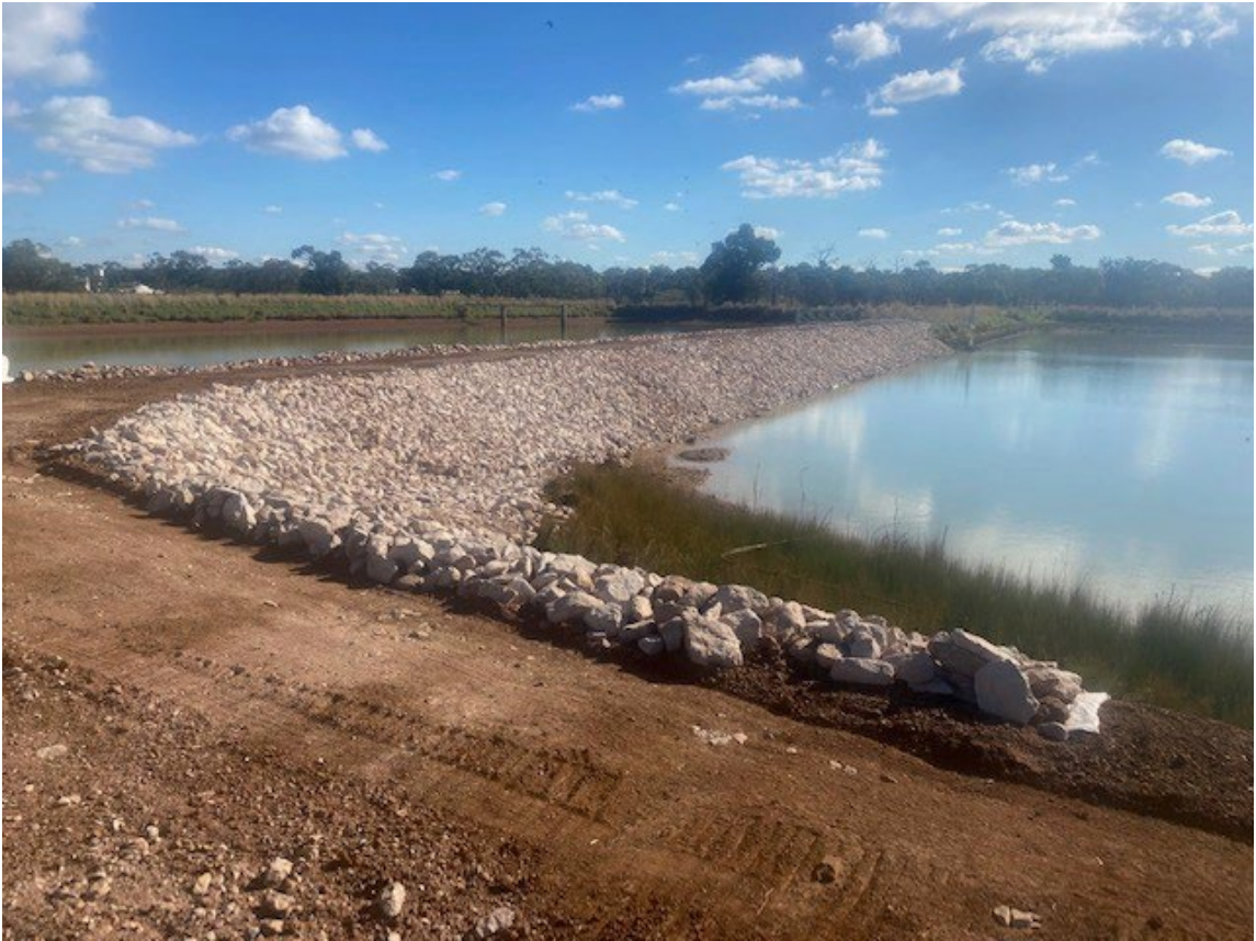
Rankins Springs Billings Road Dam Rehabilitation
