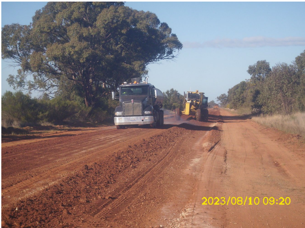
Added water with blade work – 10 August 2023
