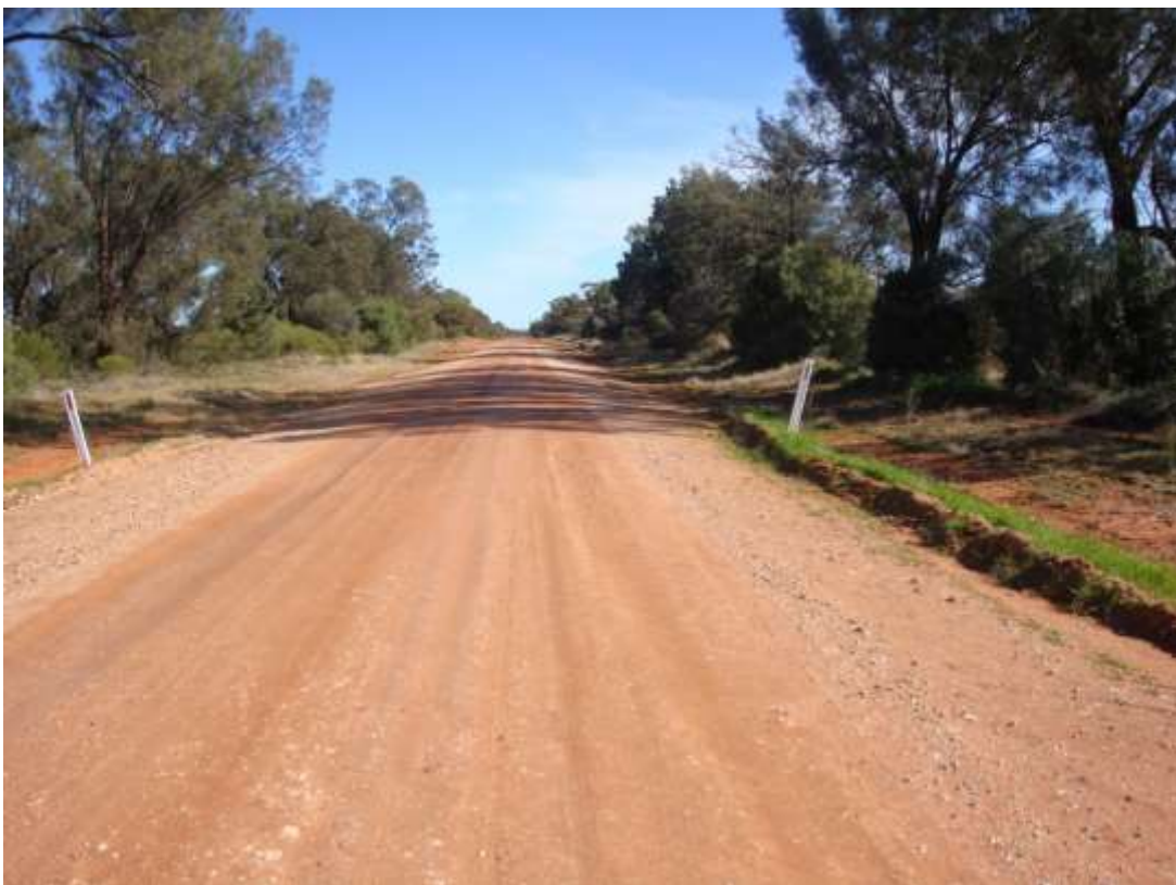
Photo 3: Arcadia Lane. Unsealed road with a constituent of mainly loam material. Historically, roads that have these types of material respond well to maintenance grading using optimum moisture either naturally or manually applied and compaction. Polytahr has thus far displayed good characteristics in maintaining the pavement and shape of the road thereby allowing for a more comfortable journey.
