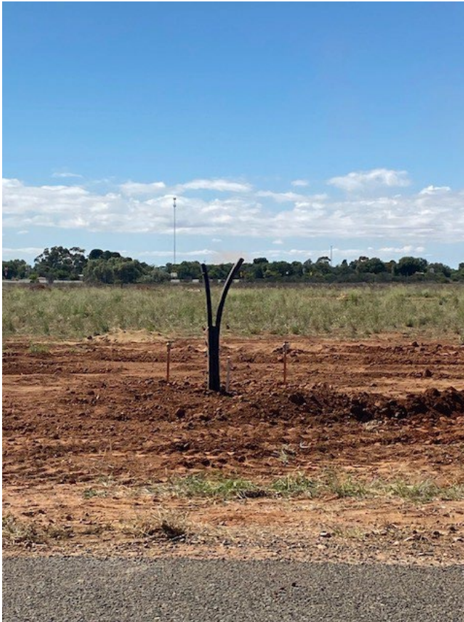
Hillston Subdivision Works – Water Services to Individual blocks
