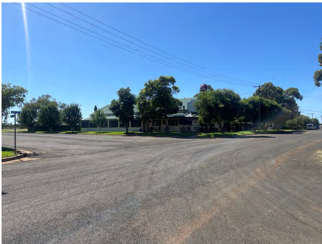
Photograph 7: Black Stump Hotel. Photograph taken facing south east.
