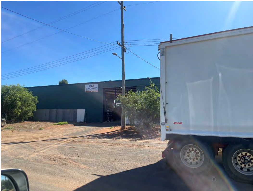
Photograph 13: Crowe's Mechanical and Engineering workshop. Photograph taken facing east.
