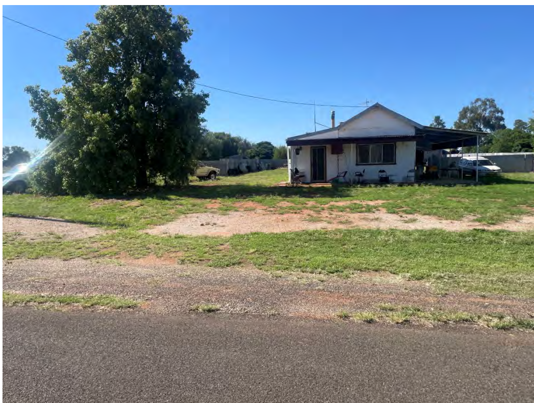
Photograph 2: Typical house in Merriwagga.
