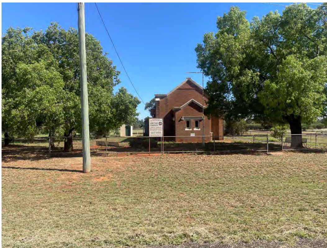
Photograph 12: Uniting Church. Photograph taken facing north.
