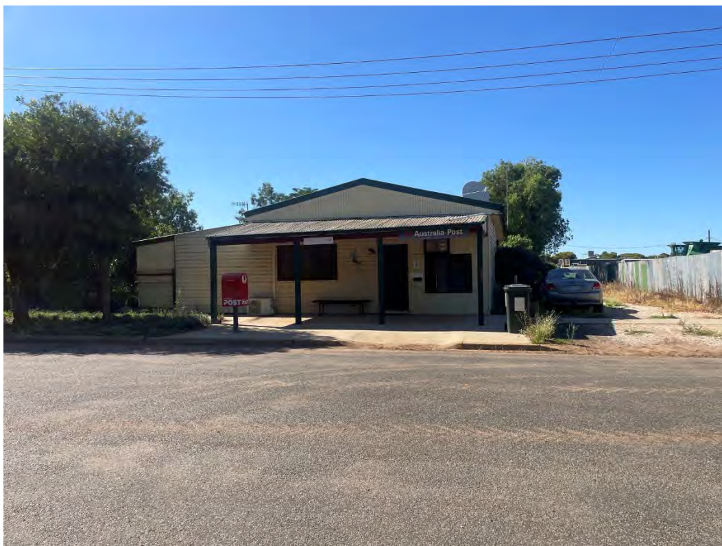
Photograph 10: Post office. Photograph taken facing south.
