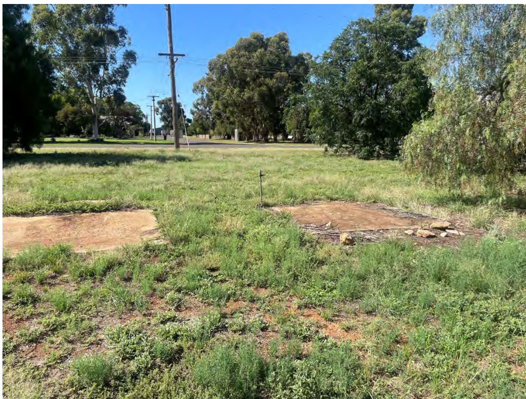
Photograph 15: Concrete pad at the former Morris & Co motor garage site. Photograph taken facing south.
