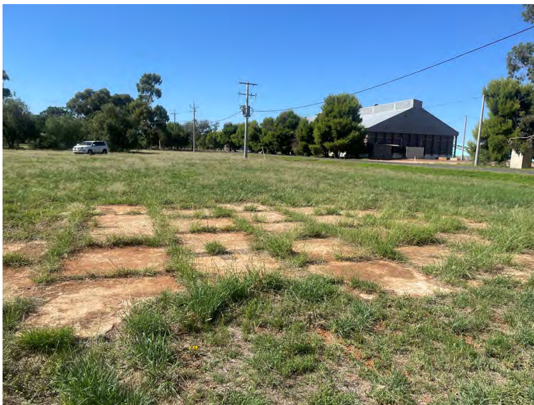
Photograph 17: Concrete pad at the former Morris & Co motor garage site. Photograph taken facing south west.
